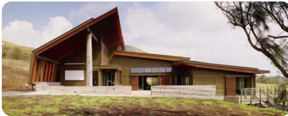
The Energy Lab, Kamuela Hawaii
