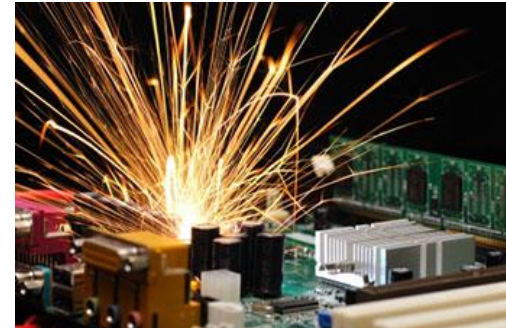
Failing capacitor Source: clemson.edu
