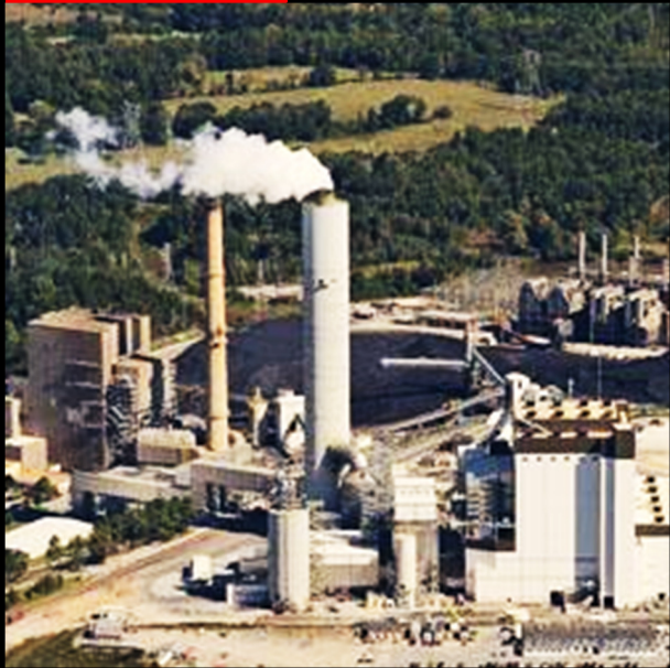
COAL POWER PLANT
