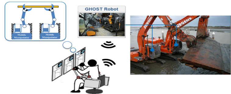
Remotely controlling multiple unmanned excavator robots
